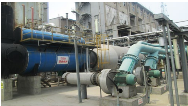
DNCC installed a new incinerator to burn waste water and gas from the production process.
